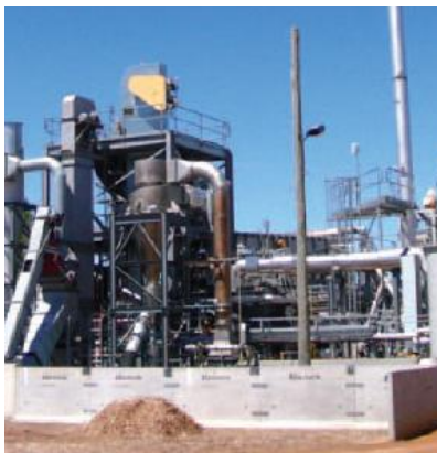
A biomass-fired power plant
