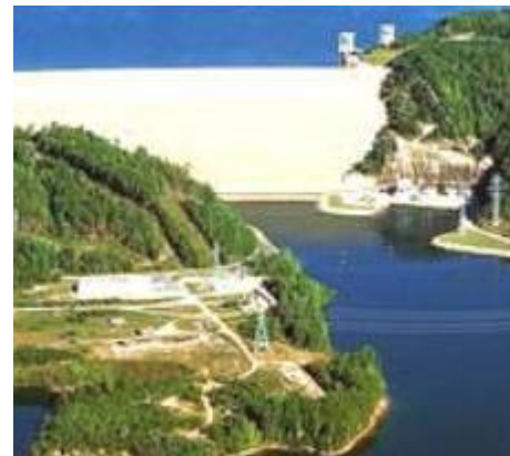
A pumped hydro facility
