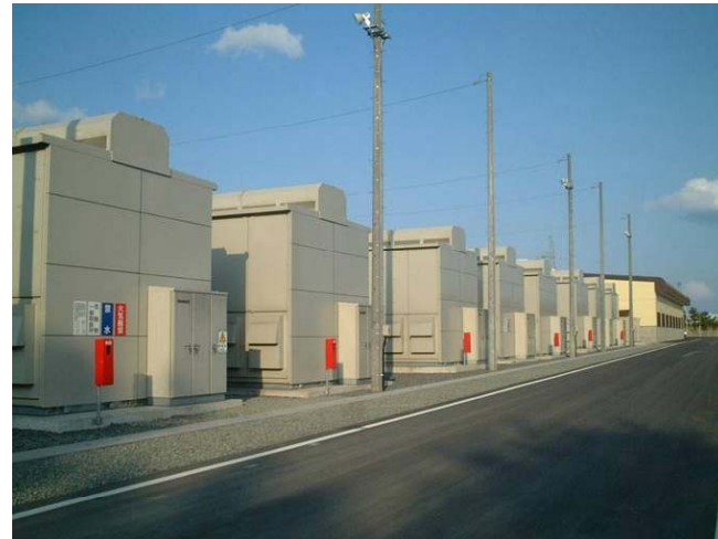
34MW NAS Battery
