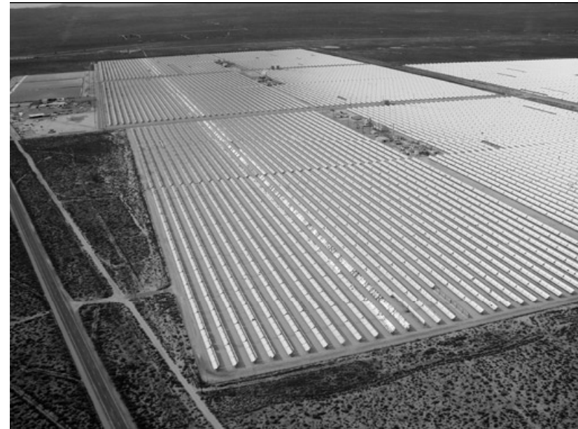
Kramer Junction, Californie, 150 MW
