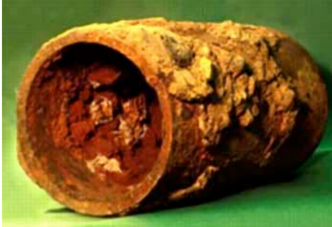
Sludge / corrosion tuyauteries
