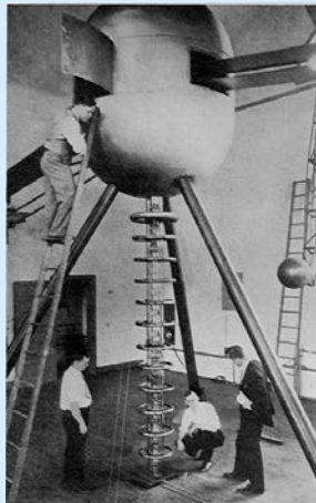
PLATE 24 The Carnegie Institution's two-meter Van de Graaff. Dahl is on the ladder. Tuve in the room. The business end of the discharge tube, deflecting magnets, and pumps are under the floor. Tuve, Halstad, and Dahl. PR. 49 (1935), 322.
