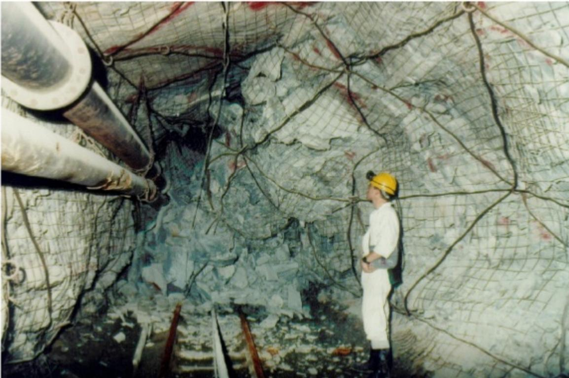
Aftermath of a rockburst in a deep-level tunnel showing complete tunnel closure. The energy released by this event is **equivalent to magnitude  $M = 3.4$  earthquake**.
