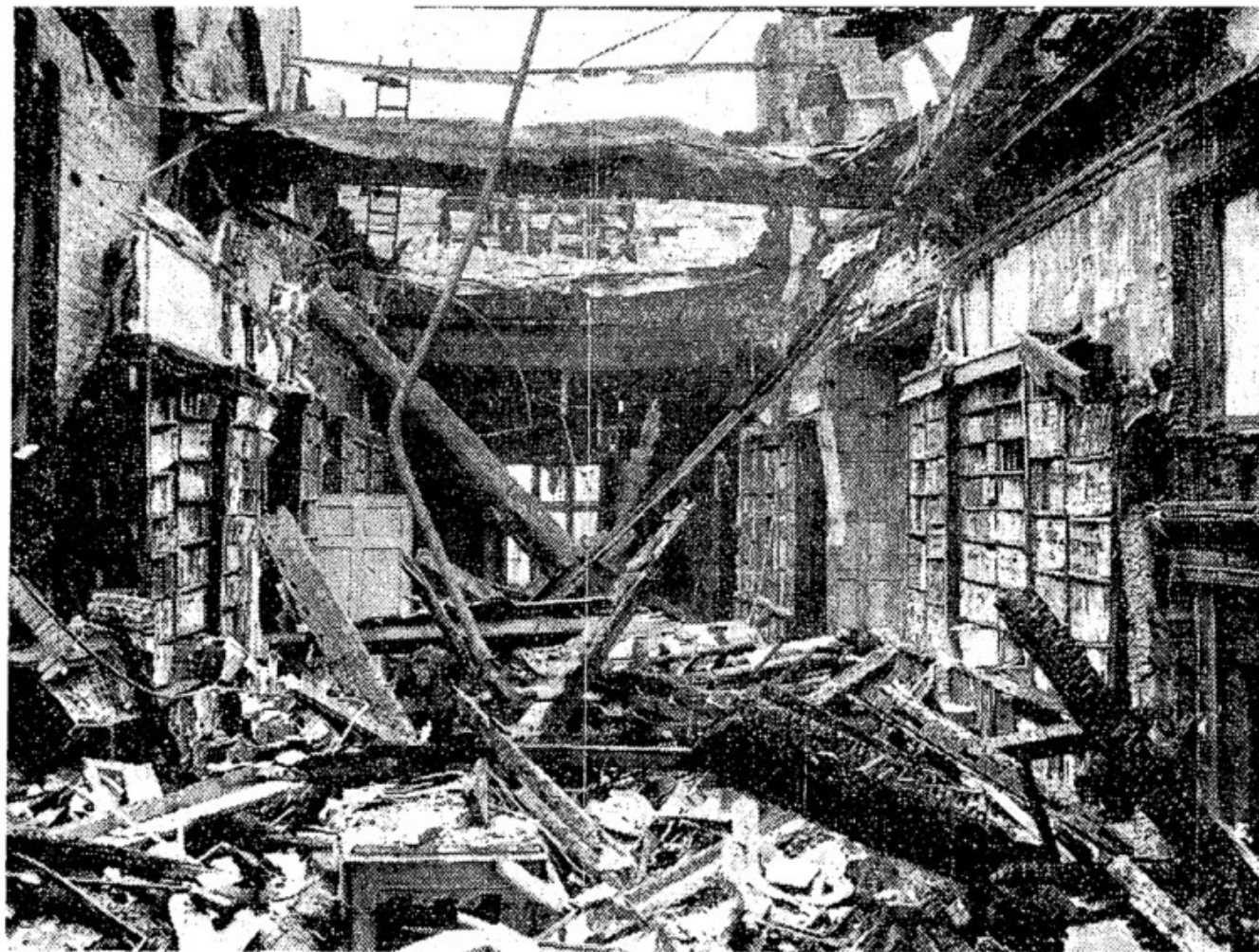
Charred timbers and burned books line the once-mellow interior
